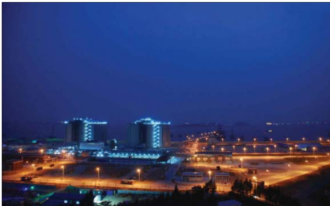
CNOOC Fujian LNG Co. Ltd. awarded a contract to CB&I for storage expansion at the 2.6 million-tonne/year LNG terminal in Fujian Province, China. CB&I will design and build two additional 160,000 cu m, full-containment LNG tanks. Photo from CB&I.
